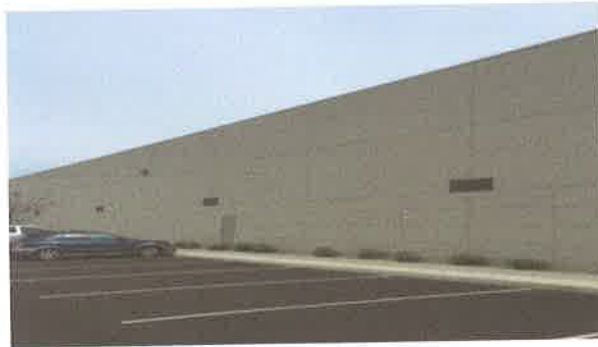
Example of poorly articulated industrial building
