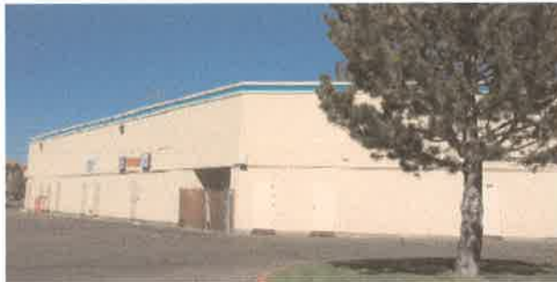
Example of poorly articulated wall facing a public street.
