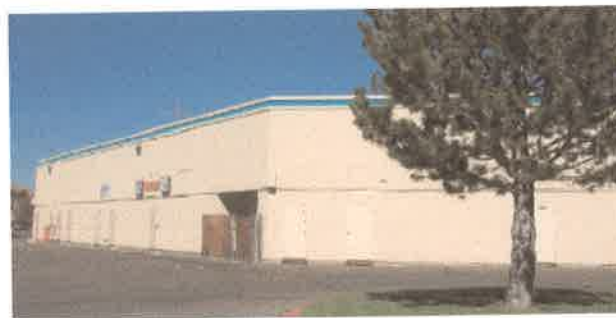
Example of poorly articulated building wall.
